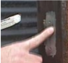
Figure 6-10. Apply rust inhibitor
