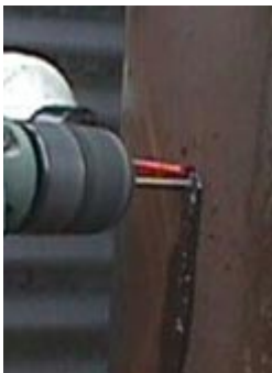
Figure 6-6. Drill mounting hole
