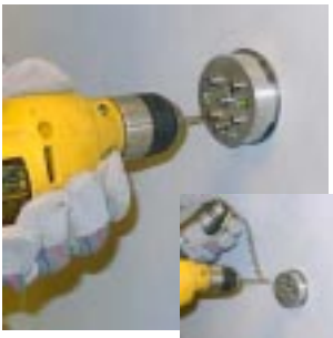
Figure 5-21. Drill Mounting Holes
