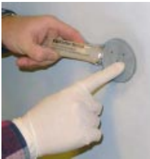
Figure 5-25. Apply rust inhibitor
